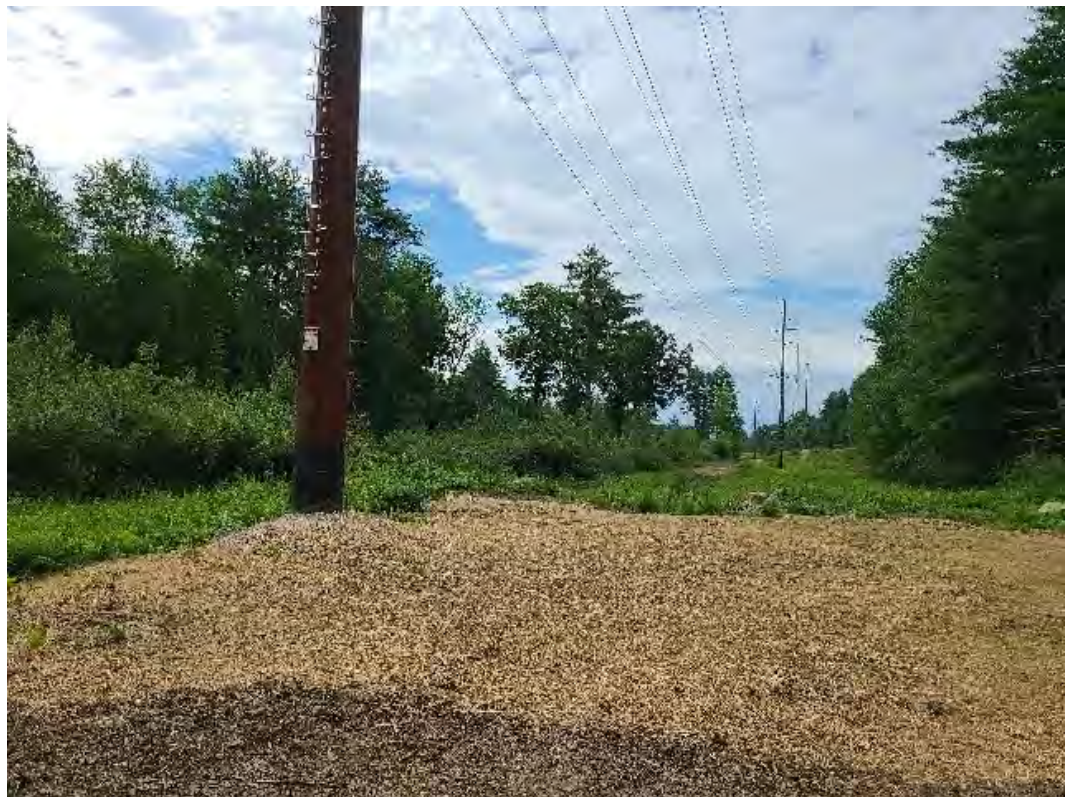
Fig 8: Str. 39 area restored. Viewing south. (07-13-20).
