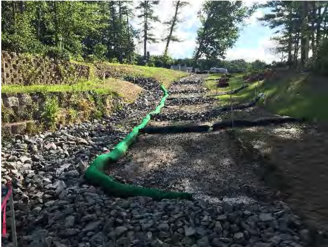
Fig 17: Temporary BMPs on slope above manhole at Gundalow Landing/east side of the bay. Viewing northeast. (07-15-20).
