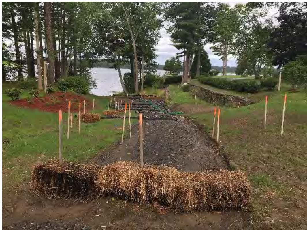
Fig 10: Slight sediment build up on BMPs on slope above manhole at Gundalow Landing/east side of the bay. Viewing west. (07-14-20).
