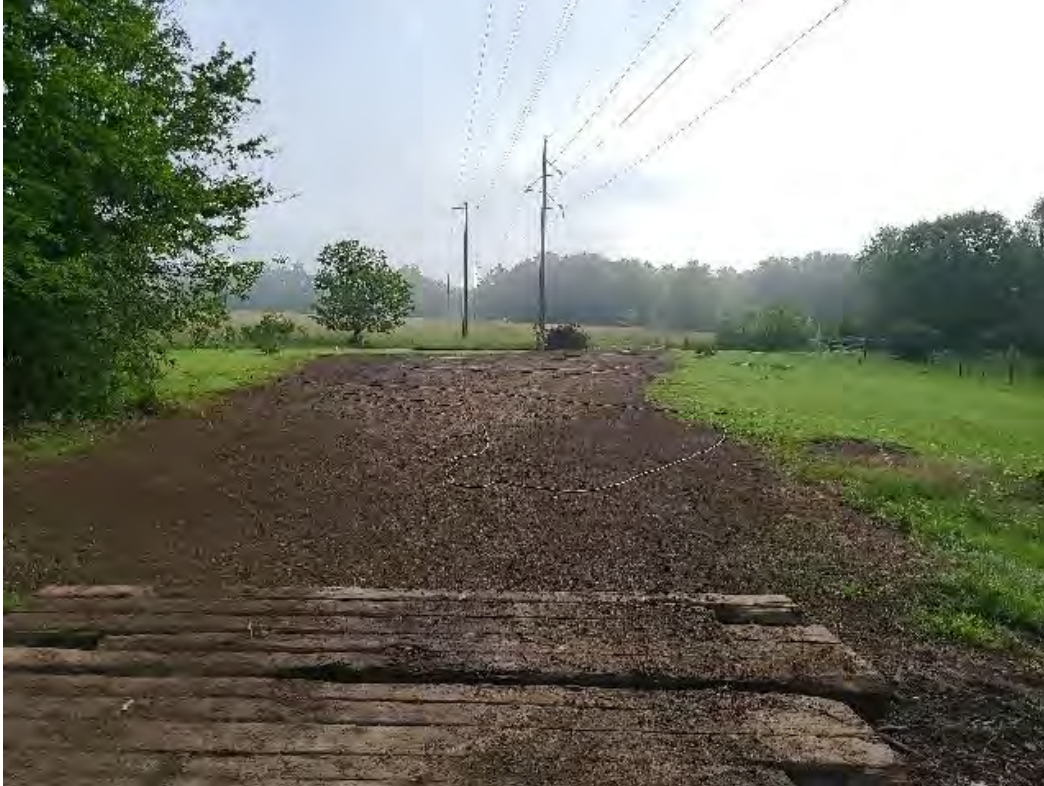
Fig 3: Restored access road between Strs. 109 and 110. Viewing northeast. (07-09-20).
