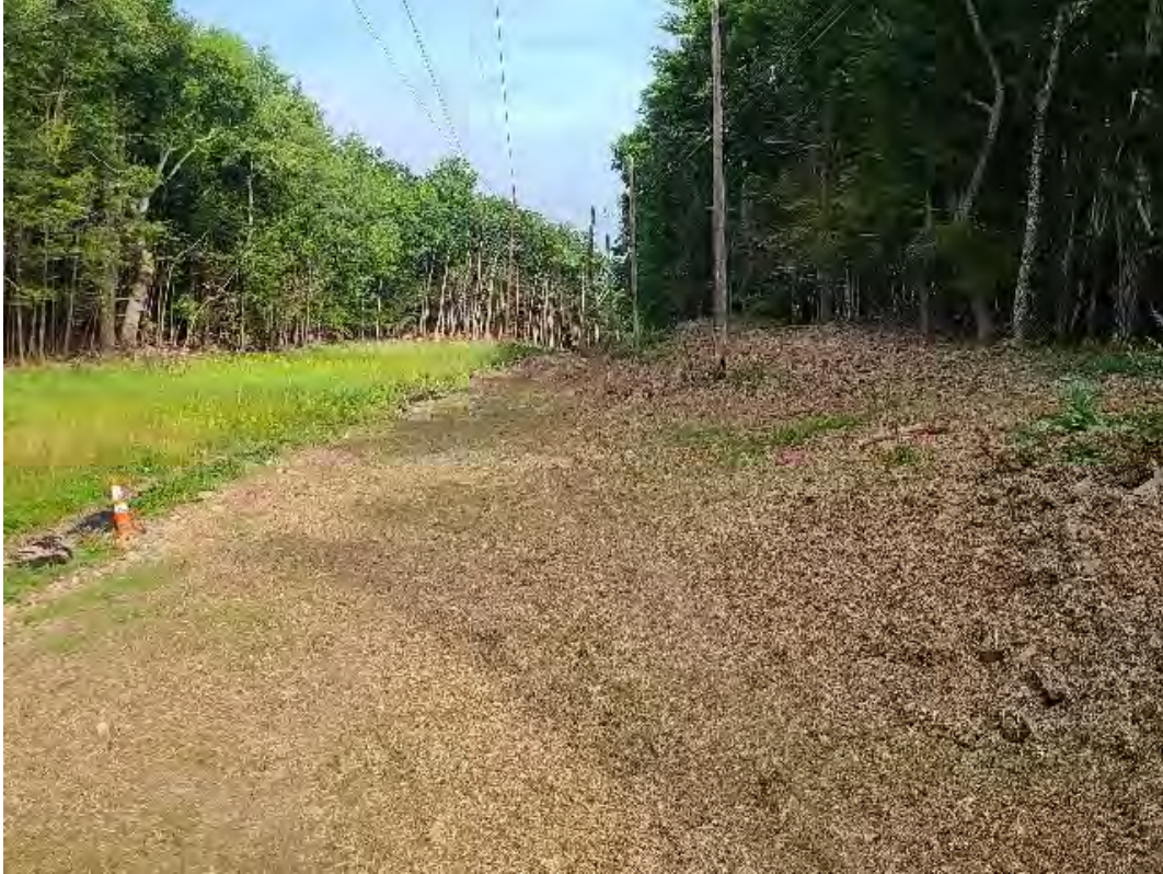
Fig 5: Slight germination on access road between Strs. 97 and 98, post restoration. Viewing west. (07-10-20).
